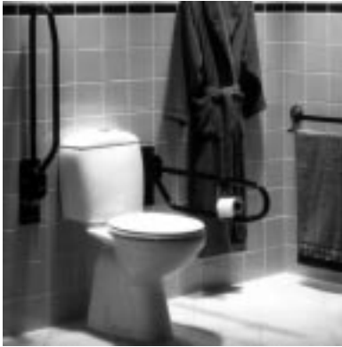
Fig. 10 Pivoting bars offer a wide range of accessibility options (photo from Linido USA)
