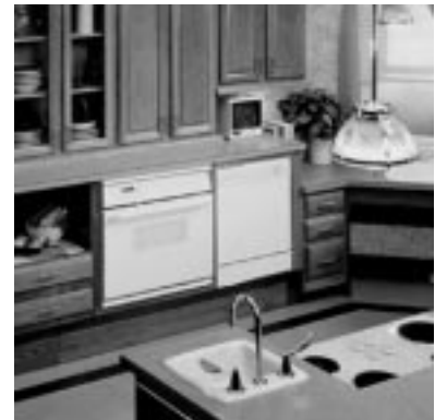
Fig. 4 Multiple counter heights enhance accessibility in the kitchen (photo by MJ Peterson)
