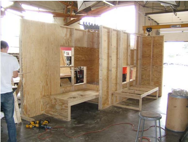
Full scale mockup of part of the cabin under construction.
