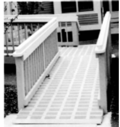
Fig. 11 Ramp with non skid surface (photo by Deckgrates)
