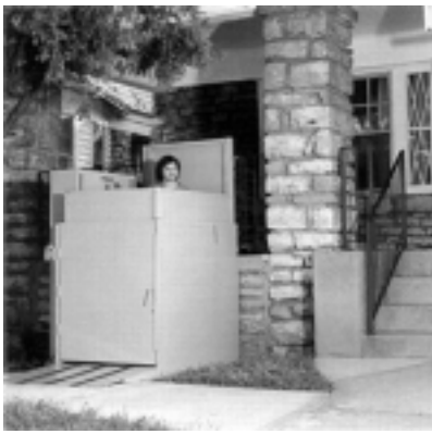
Fig.19 Lift platform with barrier (photo by Porch-Lift)
