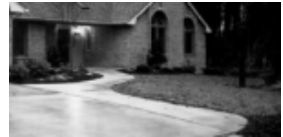
Fig.16 "Landscape ramp" eliminates the needs for steps (photo from HUD)
