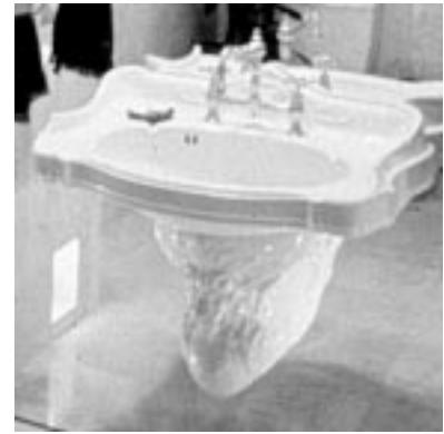
Fig 9. Sinks with built in shrouds reduce the risk of injury from hot pipes (photo by MJ Peterson)
